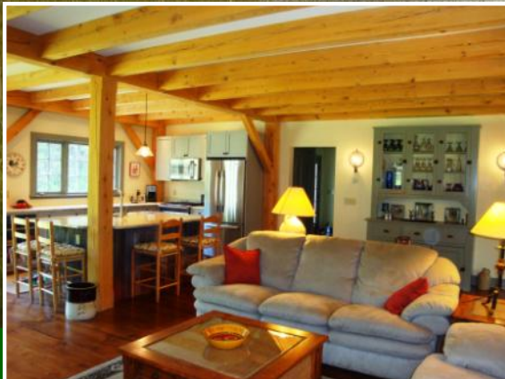
Custom timber frame Great Room has true mortise & tenon joinery, 9' ceilings and warm wide pine flooring.
